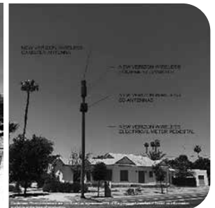
Coronado Road/5th Avenue: As stated earlier, this site is still pending. The picture shown is a possible structure that may be constructed as shown. We are doing our best to move this across to the SE corner of the area, but face multiple challenges with APS, drainage, and easement space.
