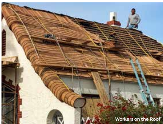
Workers on the Roof
